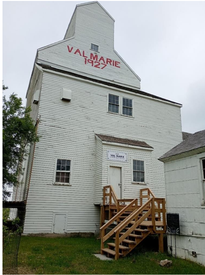
Figure 6.5: The Val Marie elevator. Photo by author.
