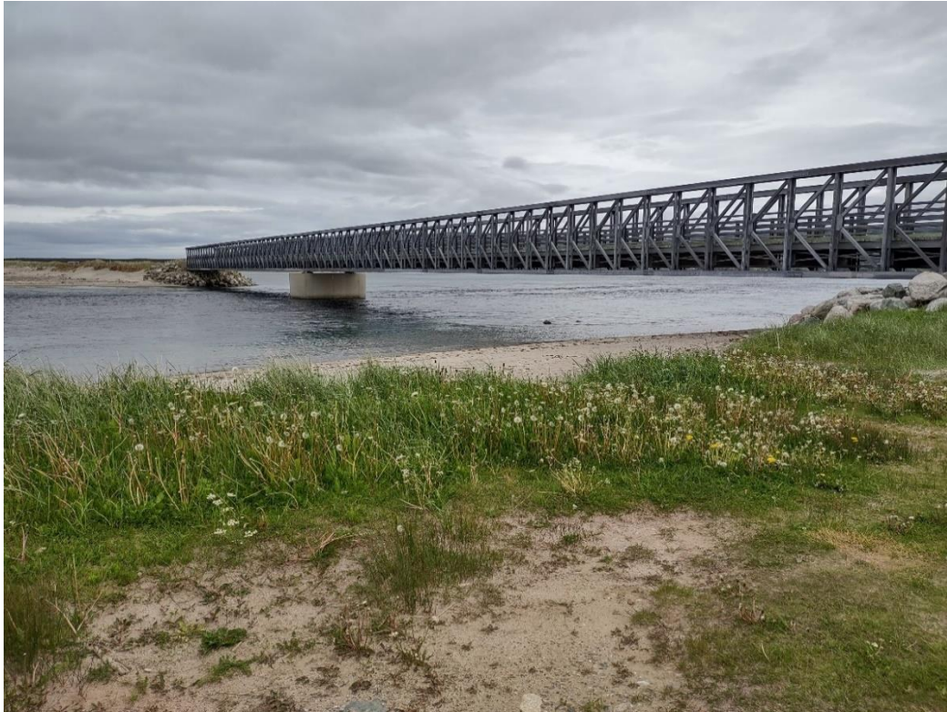
Figure 1.2: The Bailey Bridge at Searston Beach. Photo by author.
